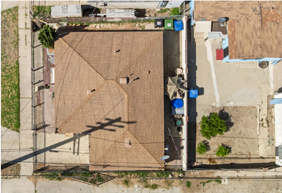
Aerial of Roof
