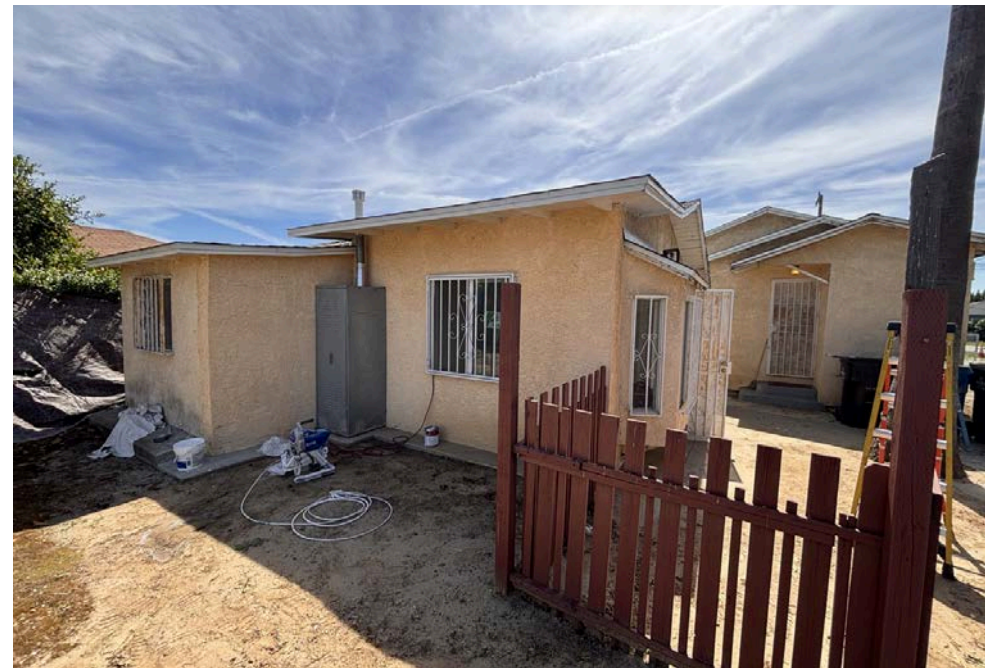
Bonus Room Structure
