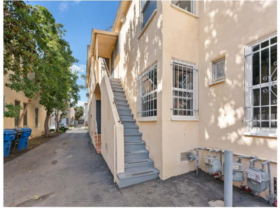
Stairs Leading to 2 nd Story Units
