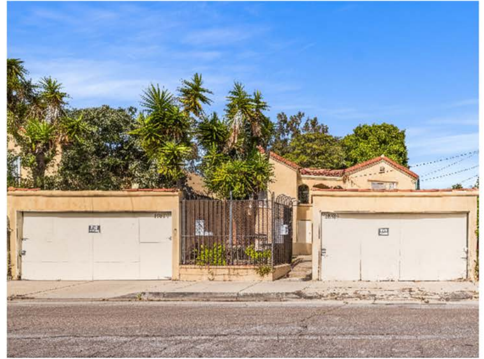
Garages & Back of Property - Street to Street Lot
