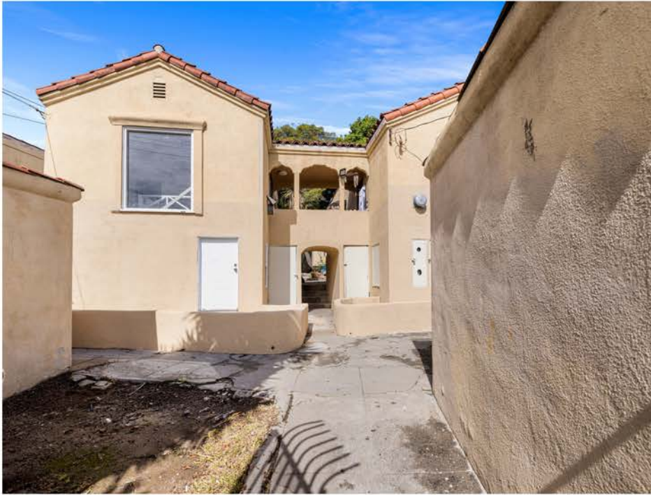
Doors Access Lower Level of Back Units & Storage
