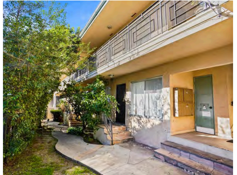
Bottom Units and Tenant Mailboxes
