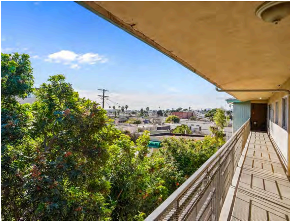
View from 2 nd Story Facing West
