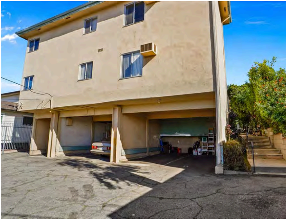
Soft Story Retrofitting & Foundation Work Done in 2018
