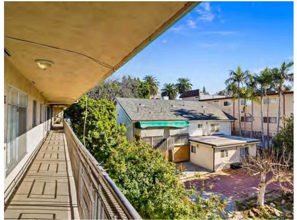
View from 2 nd Story Facing South East
