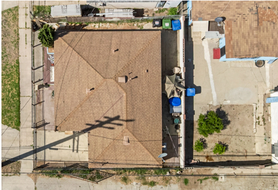
Aerial of Roof
