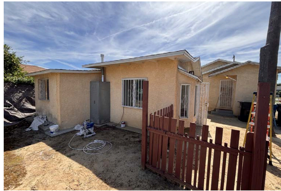
Bonus Room Structure
