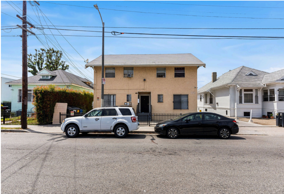
Front of Property
