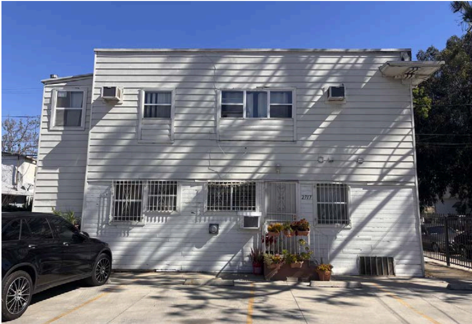
Front of 4 Unit Building
