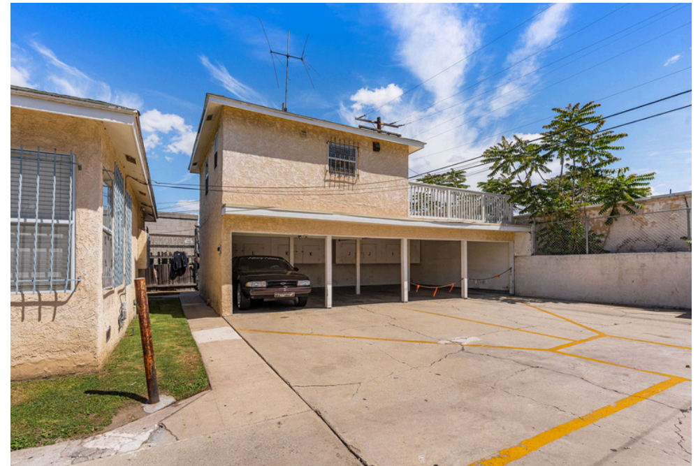
Unit 1004-B and Carports
