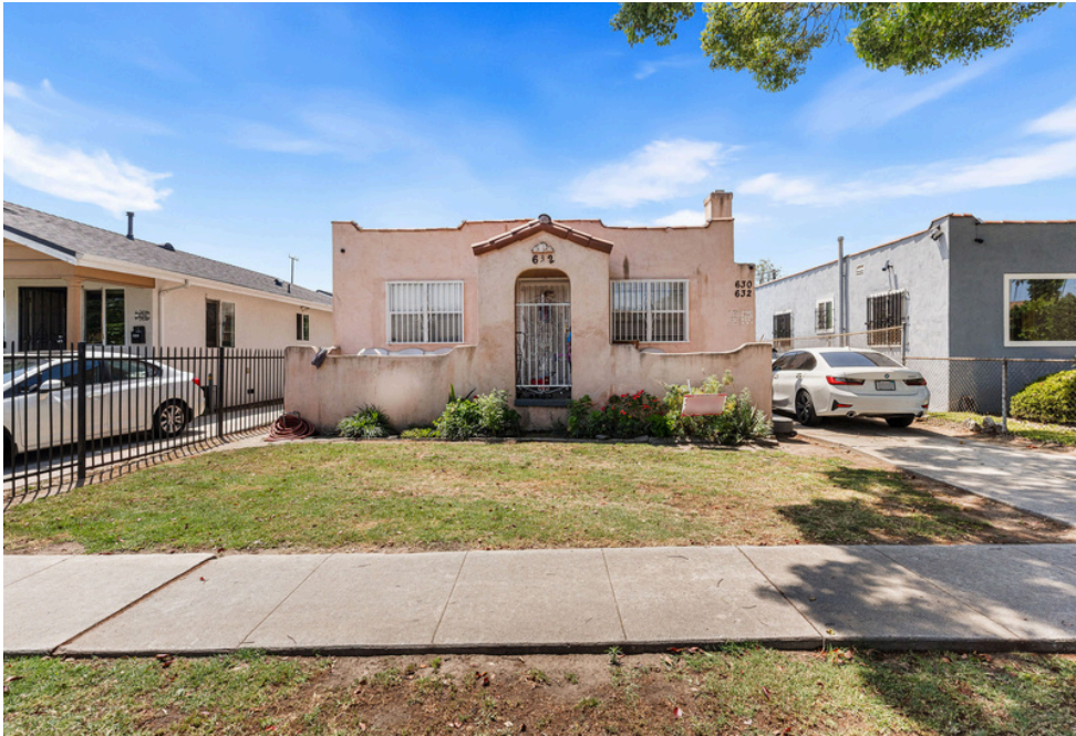
Front of Property
