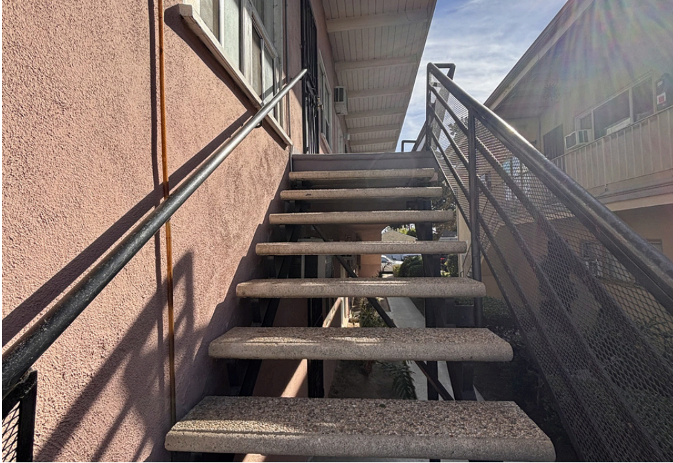
Stairs Going to 2 nd Story Units
