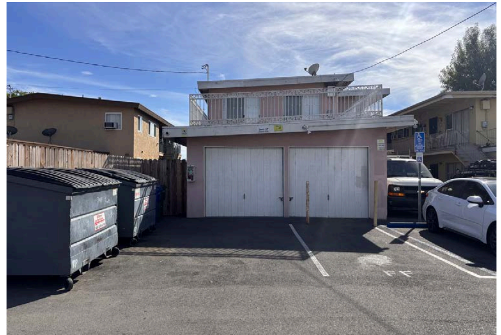
Garages and Balcony
