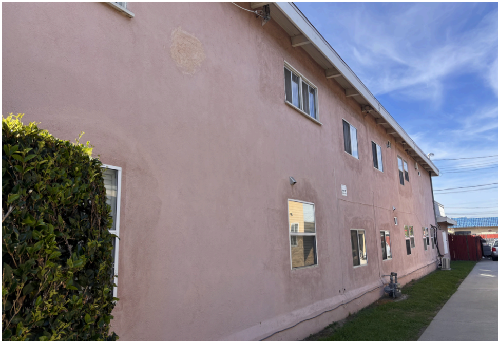
Side of Property
