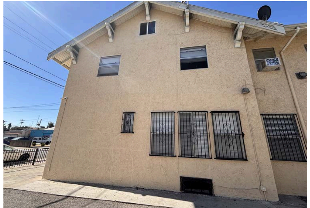
Side of Property
