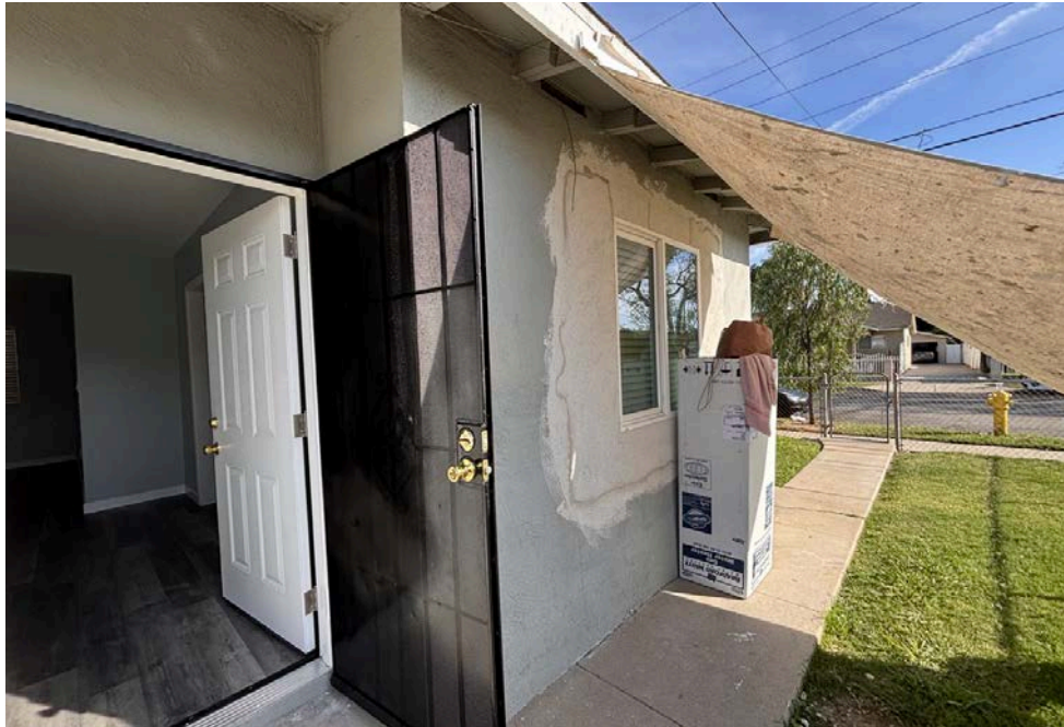
Entrance to Vacant Unit
