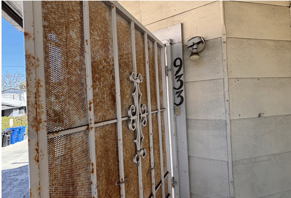
Front of 4 Unit Building
