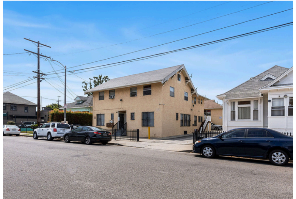
Front of Property
