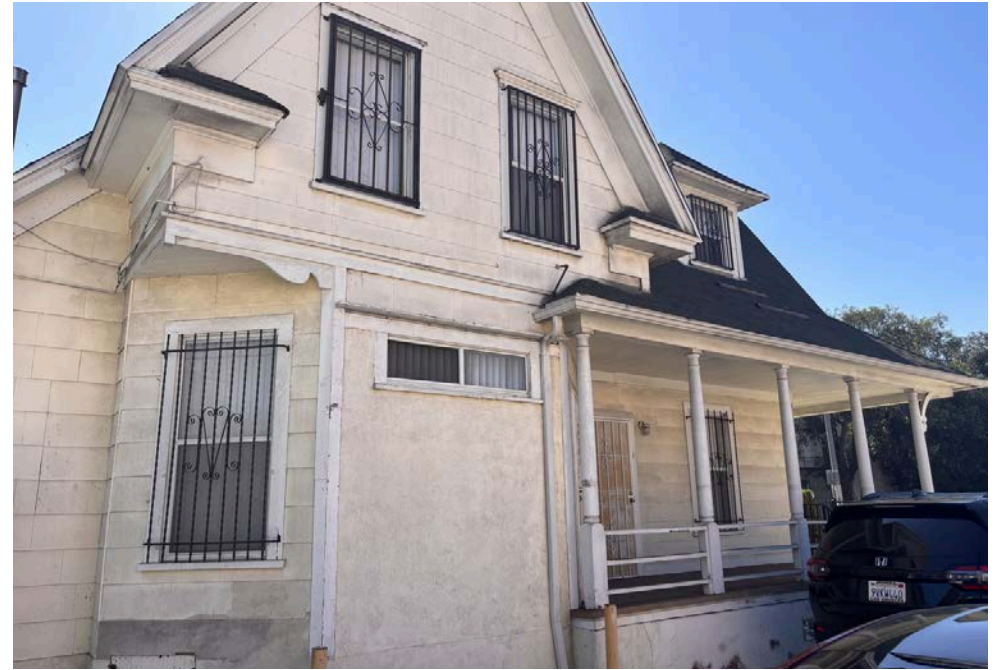
Side of Front Structure
