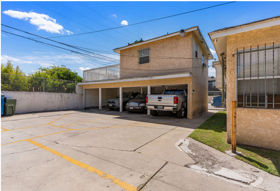
Unit 1002-B and Carports
